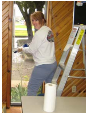
...and Melody caulks one of many windows with Carthel, the photographer
